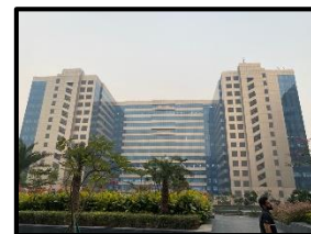
View of Tower 4, 5, 6
