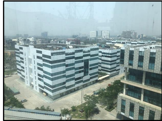
G Block of the Subject Property
