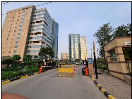
External view of Subject Property
