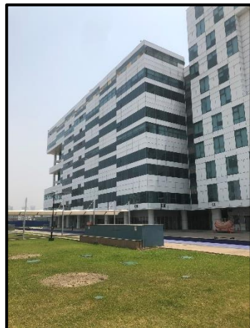
View of Tower C2
