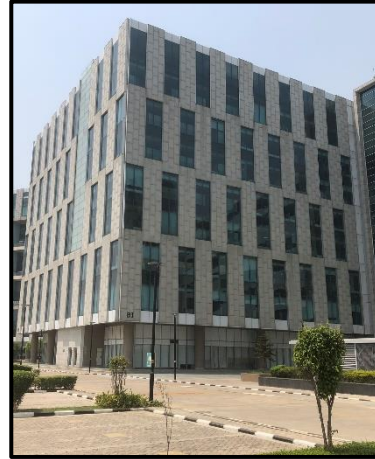
View of Tower B1
