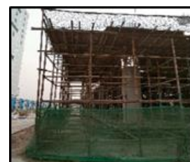
Under Construction Block 8 (Amenity Block)
