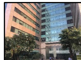
View of Tower 2 at Subject Property
