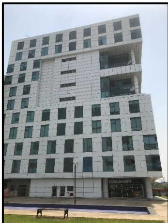
View of Tower C1
