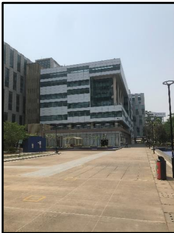
View of Tower B2
