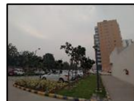
External View of Subject Property
