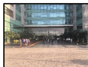
View of Tower 6 at Subject Property
