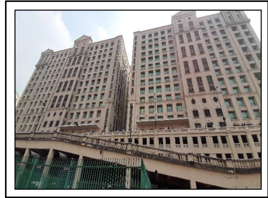
Building (A & B) – Rear View
