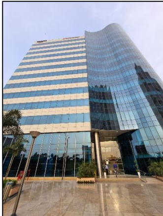
External View of Block 3
