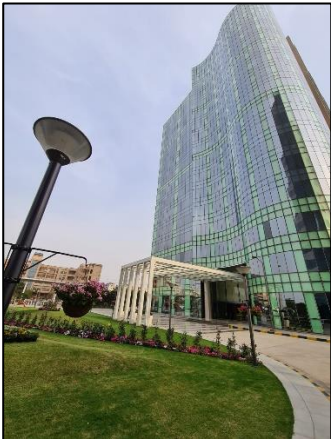
External View of Block 5
