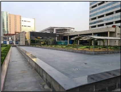
External View of Block 7
