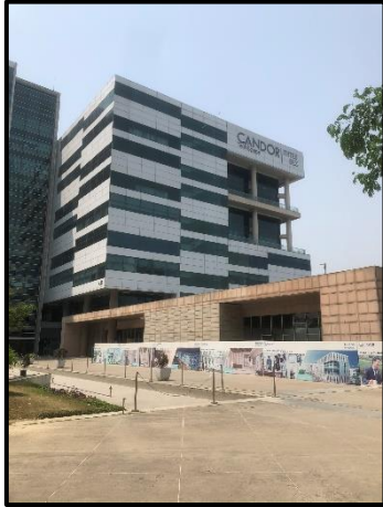
View of Tower A2
