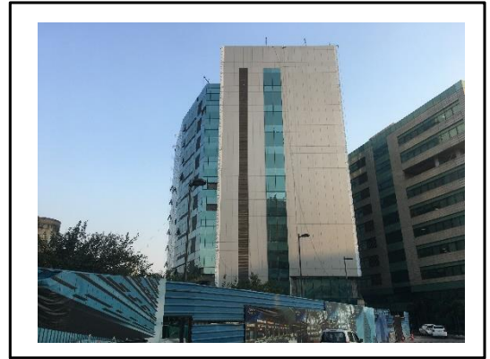
External view of under construction Tower 11
