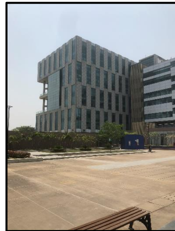
View of Tower B3
